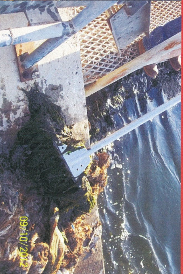
Rakes made from aluminum to clean the grates to the District's pumping plants forebays along the California Aquaduct
