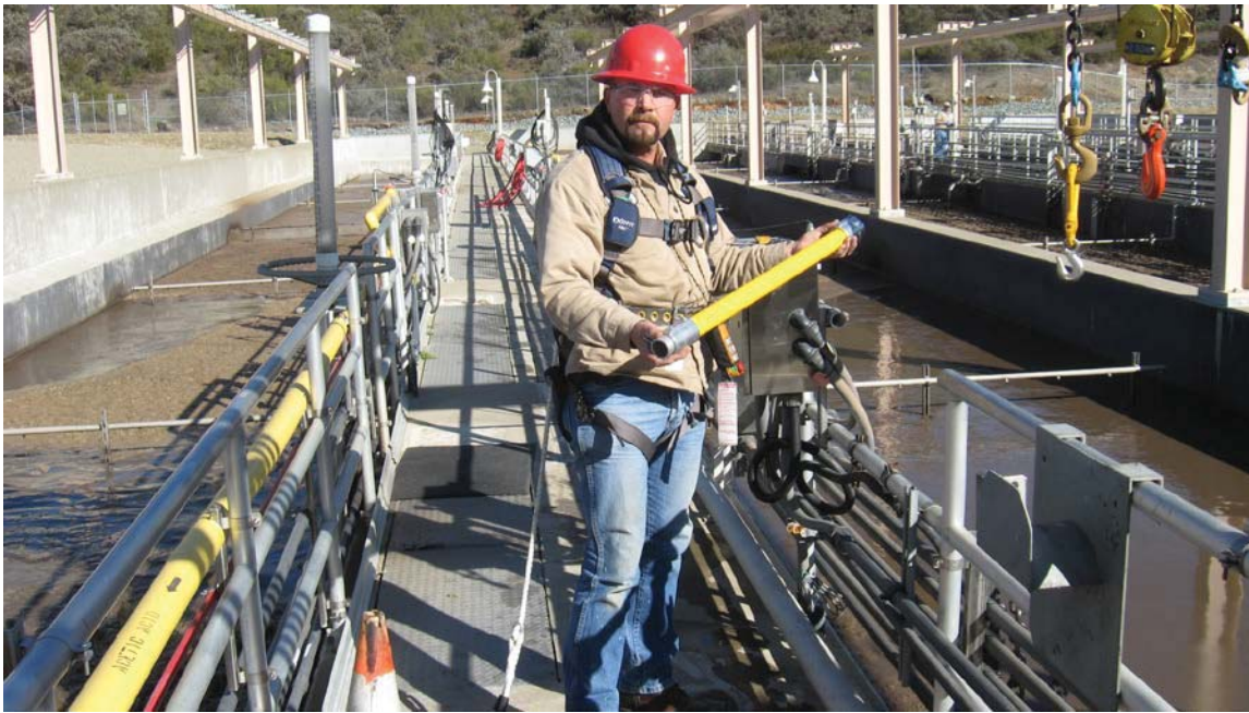
Staff removes the top guardrail that is secured using set screws.
