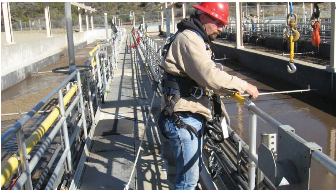
Staff attaches their full-body harness with limit-line to anchor point, and prepares to detach removable top guardrail.
