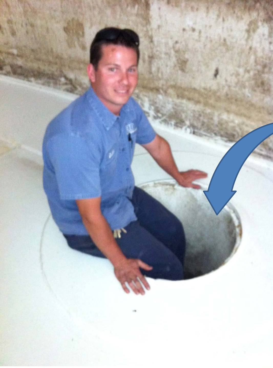
El Dorado Irrigation District Digester Discharge Pipe Cover Mike Hodges and Dustin Stoneback
